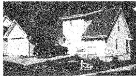
Zero step at the back on steep lot, many steps at front. (Decatur GA Housing Authority)
